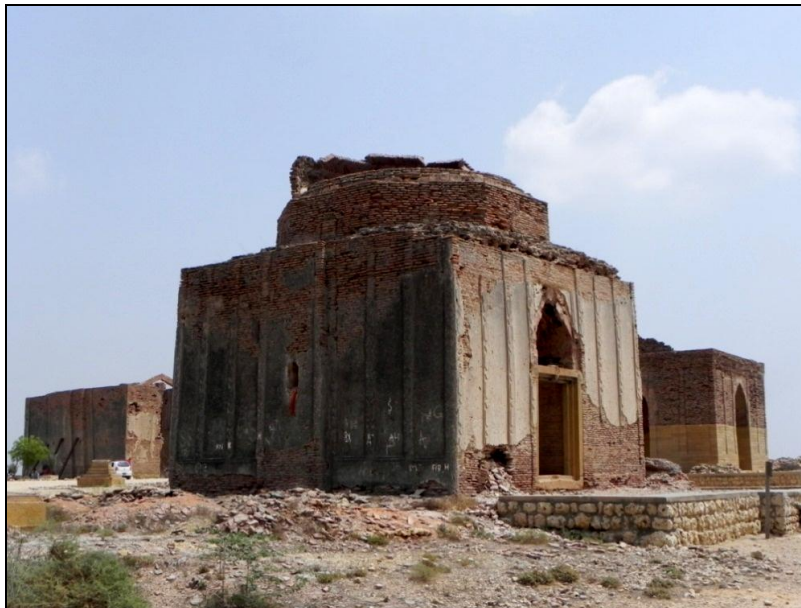
Figure 07: Brick built tombs with stone masonry till dado level, Samma period. (Taken by the author)
